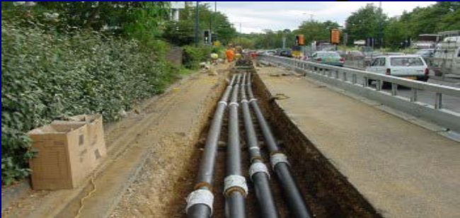
DISTRIBUTION PIPING 4 pipe system (heating & cooling)
