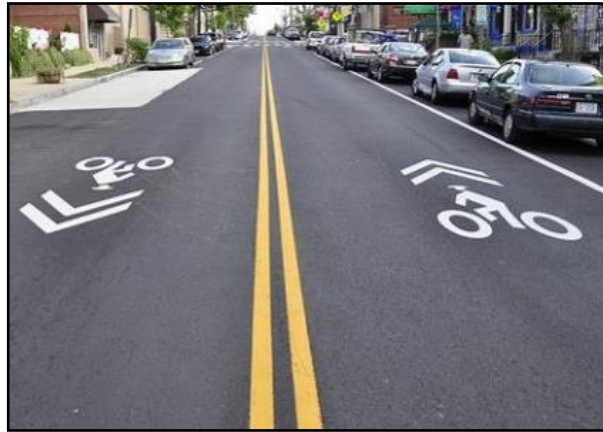
Shared Lane Marking
