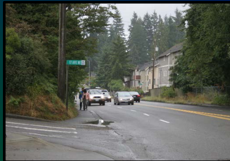
Poor sight distance and lack of left-turn management contribute to safety concerns
