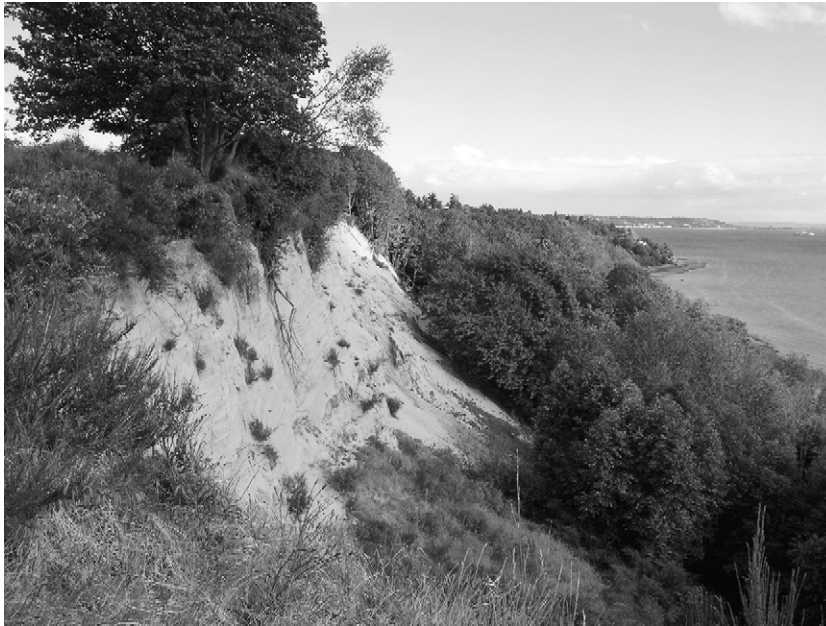
Fig. 2. Photograph showing typical vegetation in Seattle covering a landslide complex. View is toward the southeast from south of West Point (Fig. 3) on June 14, 2005. The vertical escarpment is approximately 12 m high. Photo by Jeffery Coe (US Geological Survey).
