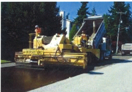
Asphalt and chips are applied to the existing pavement
