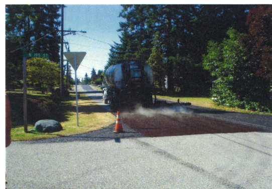
A fog seal is applied after the BST has cured
