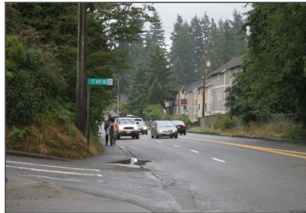
Poor sight distance and lack of left-turn management contribute to safety concerns
