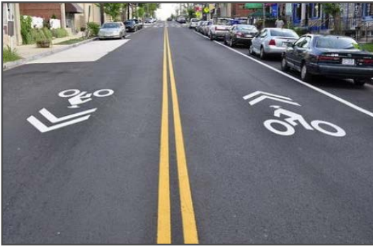
Shared Lane Marking
