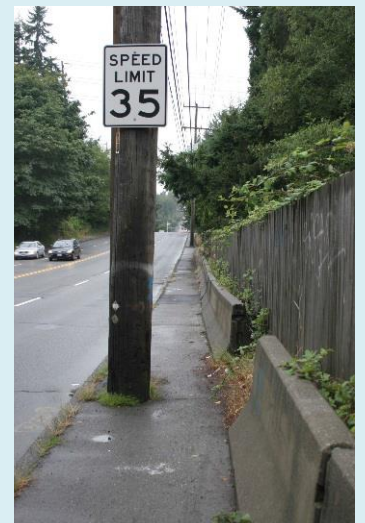
5-foot sidewalk on 145th Street
