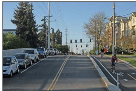
Cycle Track Curb Separated
