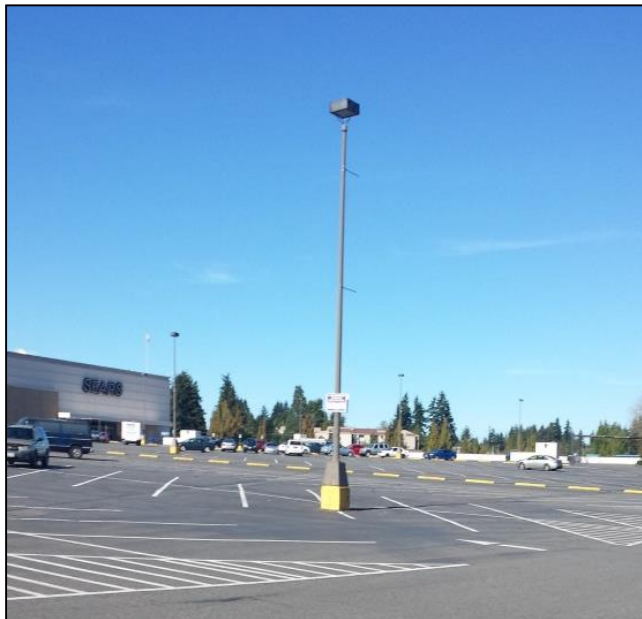
Figure 3-6. Light in surface parking lot
