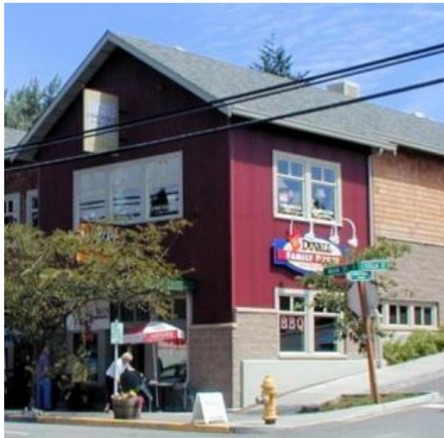
Masonry or Concrete Near the Ground and Proper Trimming Around Windows and Corners
