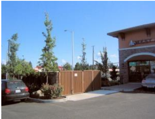
Trash/Recycling Closure with Consistent Use of Materials and Landscape Screening
