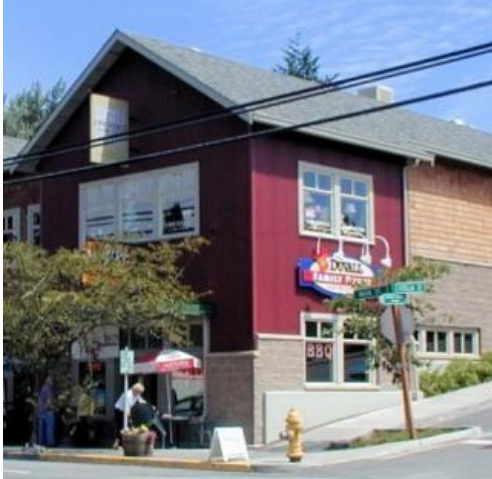
Masonry or Concrete Near the Ground and Proper Trimming Around Windows and Corners
