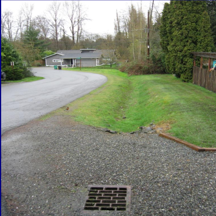
Existing Swale along Corliss Ave N
