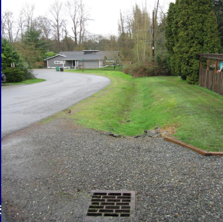
Existing Swale along Corliss Ave N
