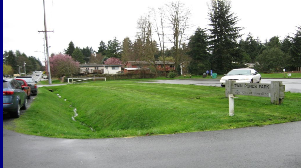
Existing Swale along 1 st Ave NE at Twin Ponds Park
