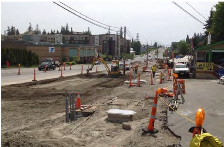
Roadway excavation and grading
