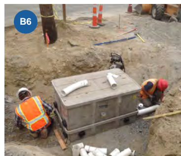
B6. Setting a Frontier vault
