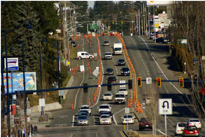
Traffic shifted to the east side of Aurora Avenue
