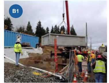
B1/B2/B3. SCL vault, cover, and lid installation
