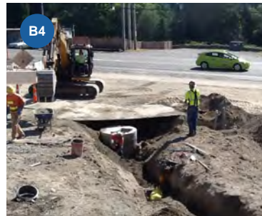
B4/B5. Installing storm drain inlets and manholes
