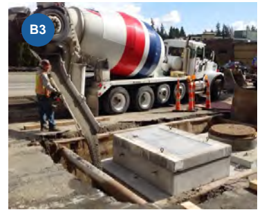
B1/B2/B3. SCL vault, cover, and lid installation
