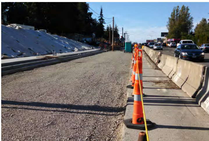
Roadbed with rock base
