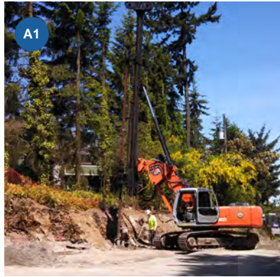
A1. Drilling for soldier piles
