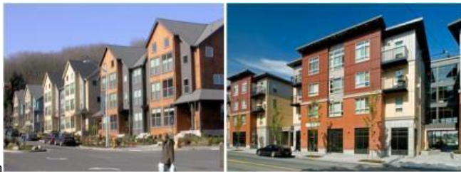
Multifamily Building Articulation
