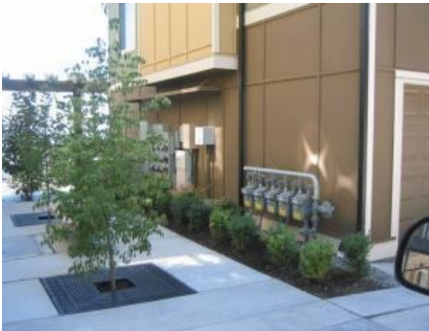
Utilities Consolidated and Separated by Landscaping Elements
