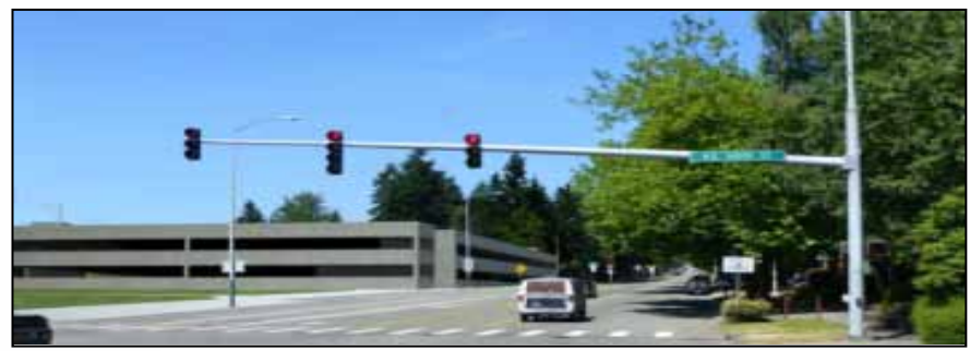
Existing and with station 5 th Avenue NE at NE 145 th Street View to the north
