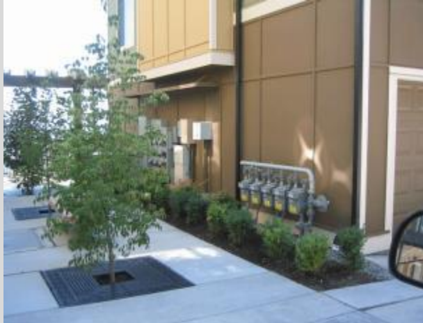
Utilities Consolidated and Separated by Landscaping Elements
