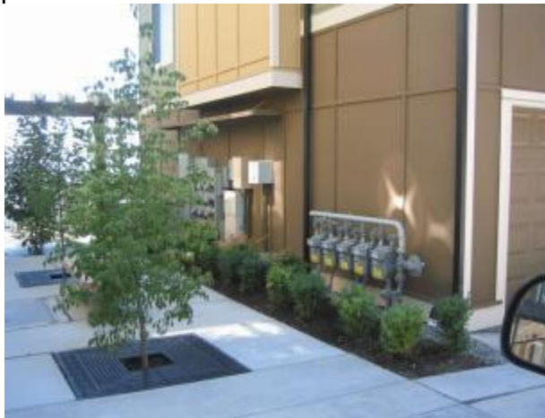
Utilities Consolidated and Separated by Landscaping Elements
