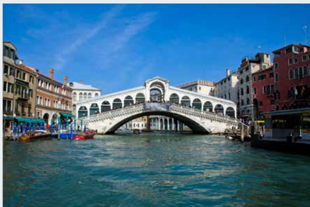
Rialto Bridge, Venice, Italy, Source: Wikipedia Commons
