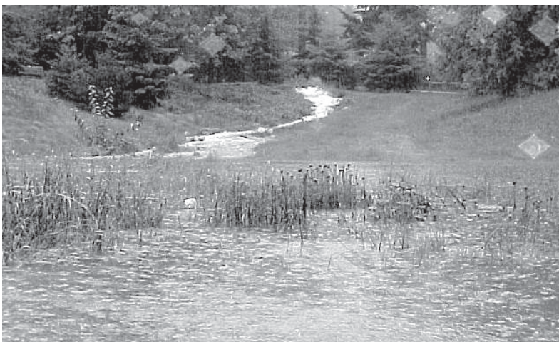
The Third Ave. NW Drainage Improvement Project includes a new stormwater conveyance pipeline and modifications to the Boeing Creek Stormwater Facility, above, to relieve long-standing flooding problems affecting approximately 20 homes.
