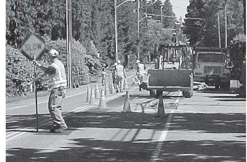
**City Road crews prepare the roadway for the annual overlay of new asphalt this summer. Cracked road surfaces are removed with a backhoe and replaced with new asphalt.**
