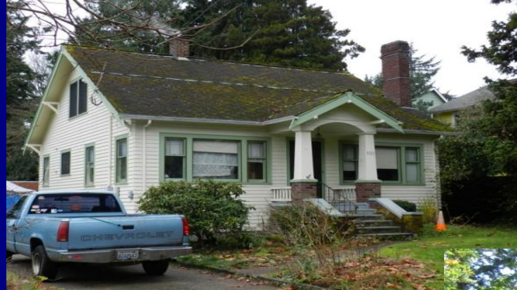
1321 N 185 th Street, 1929 added
