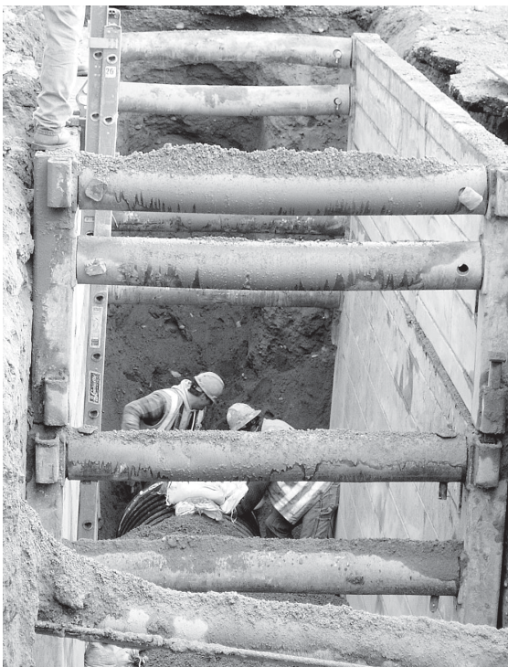
Crews work in a storm water trench near N. 160th St.
