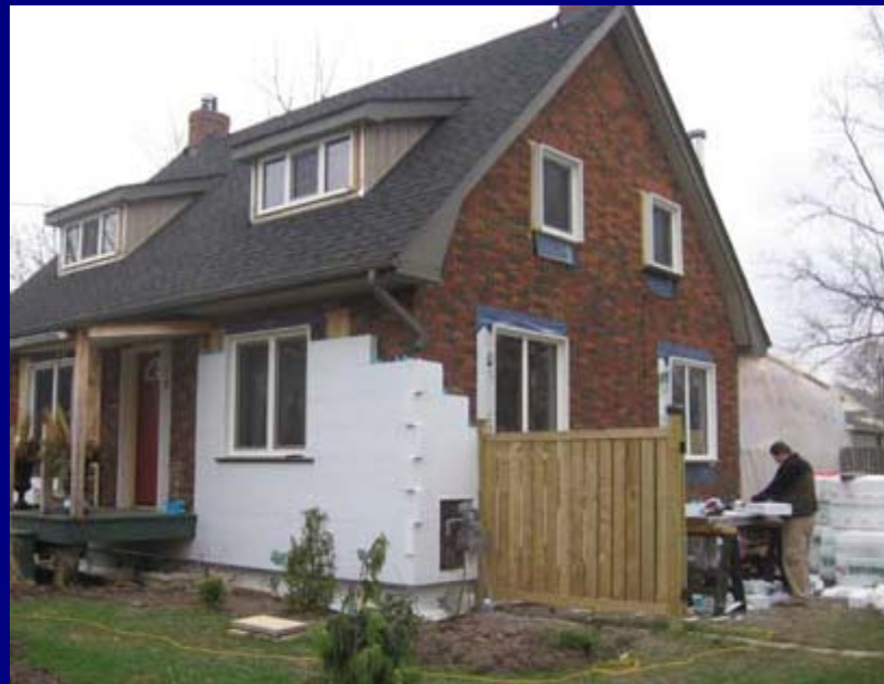
Adding Exterior Insulation on Existing House
