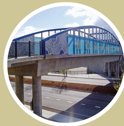
Aurora Pedestrian Bridge
