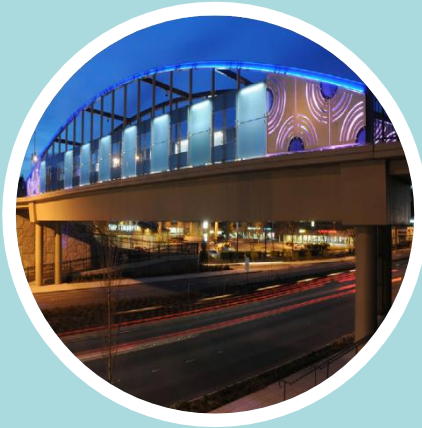
Aurora Avenue N Bridge
