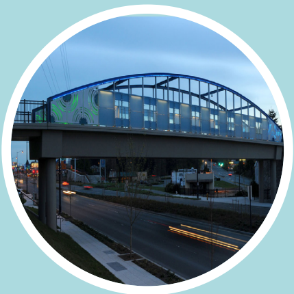
Aurora Avenue N Bridge
