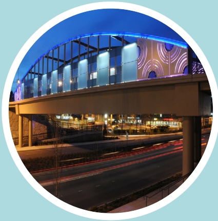
Aurora Avenue N Bridge
