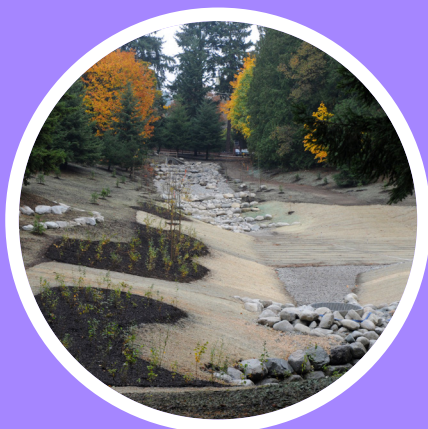
Boeing Creek Stormwater Improvements
