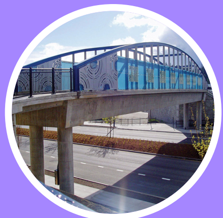
Auroa Pedestrian Bridge
