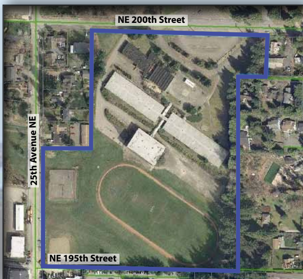
Shoreline School District's Aldercrest Annex
