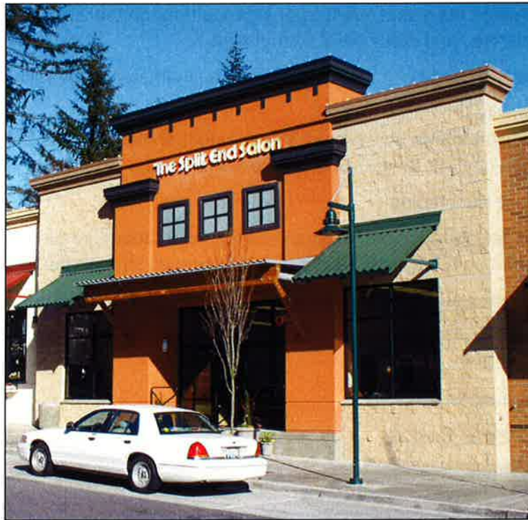
Concrete near the ground level and a variety of other surface materials on the façade.
