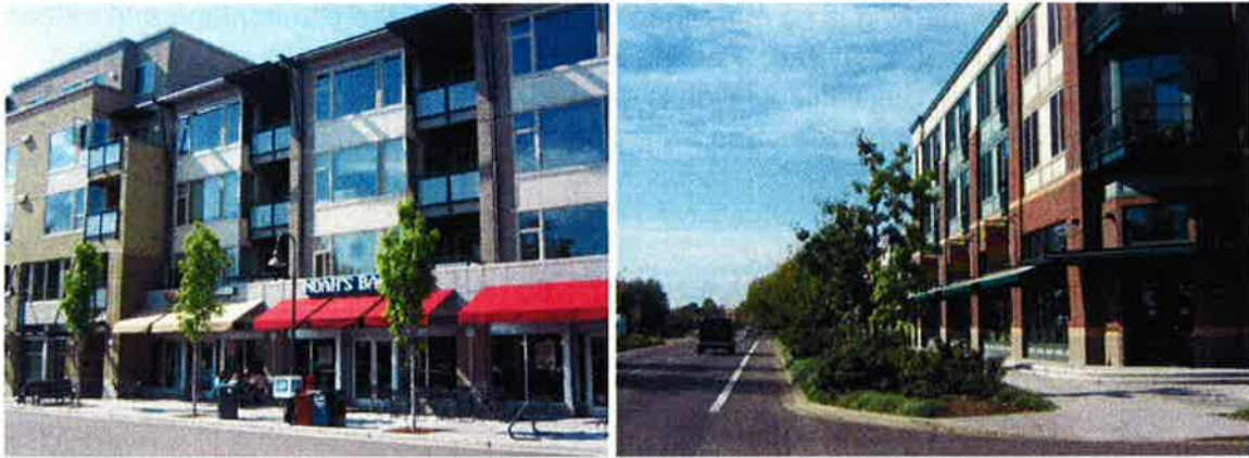
Storefront and Boulevard buildings
