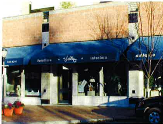
The left image uses smooth gray blocks on the vertical columns and beige split-faced blocks above the awnings. The storefront in the right image uses gray split face and some lighter, square, smooth-faced blocks below the storefront windows.
