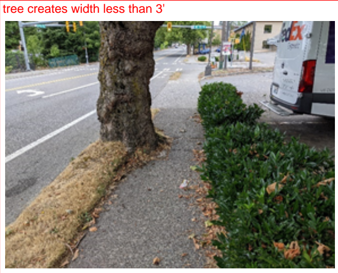
tree creates width less than 3'
