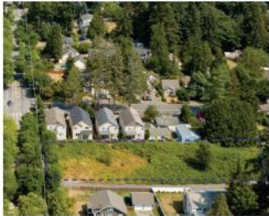
AERIAL VIEW OF SITE
