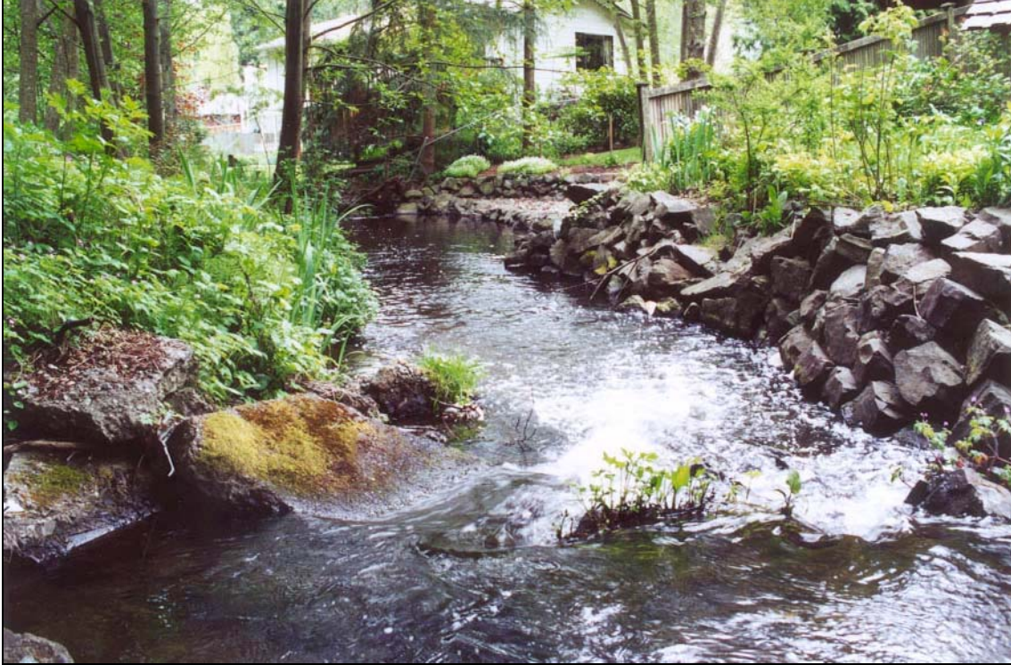
Photo 13. Pool Downstream of Culvert under Forest Park Drive on McAleer Creek
