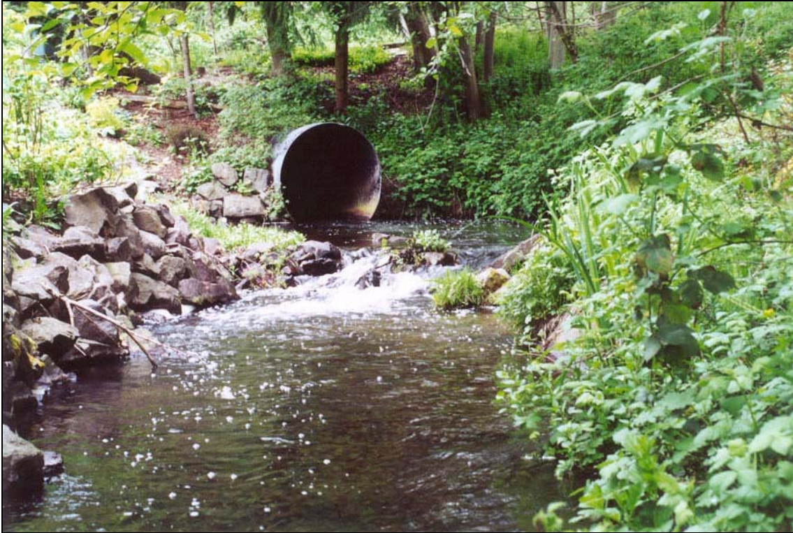
Photo 11. Culvert Under Forest Park Drive on McAleer Creek
