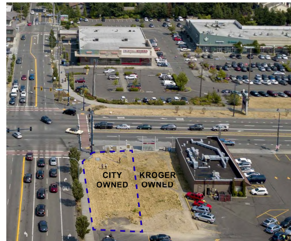
AERIAL VIEW OF SITE
