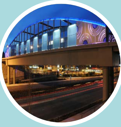
Aurora Avenue N Bridge
