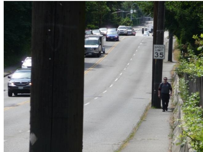
Narrow and non-ADA compliant sidewalk facilities along NE 145th Street near 10th Avenue NE
