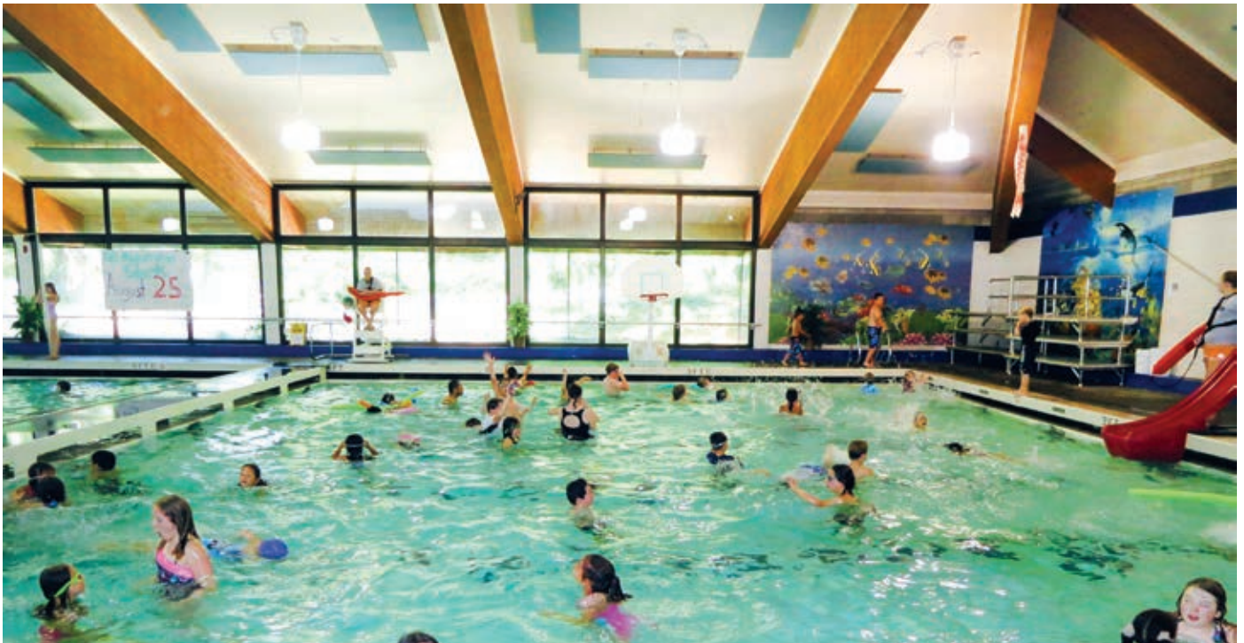
The Shoreline Pool was constructed in 1971 as part of King County's Forward Thrust Park and Recreation Bond Initiative. After 42 years of service, it now requires significant repairs in order to extend its useful life.
