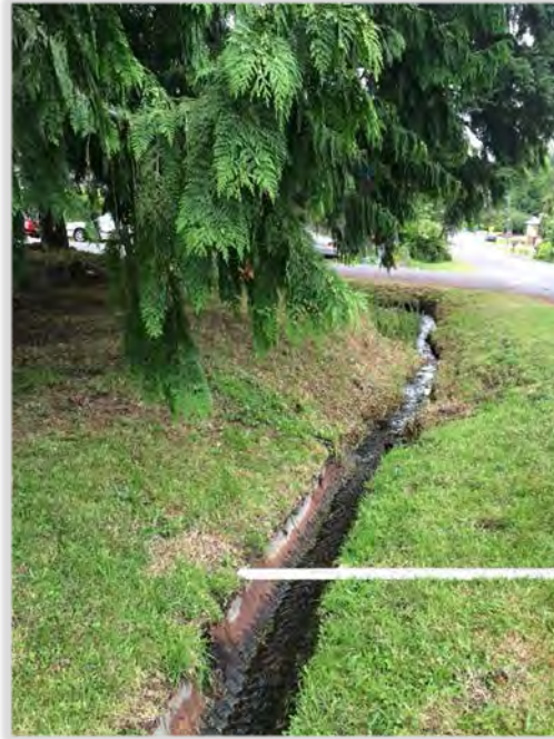
Photo 6. Example half-pipe drainage in Whisper Creek area
