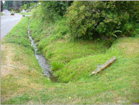
Photo 5. Example roadside drainage channel in Whisper Creek area
