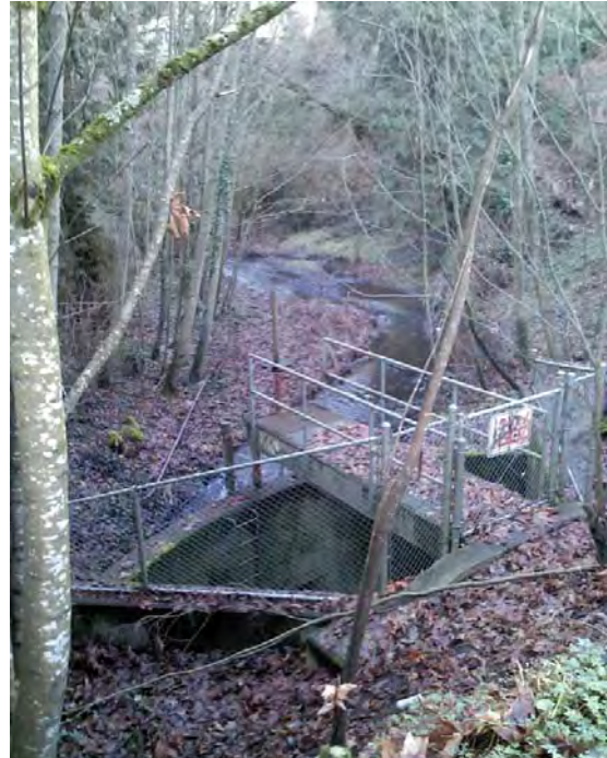
Photo 2: Flow control facility at NE 196th St.
