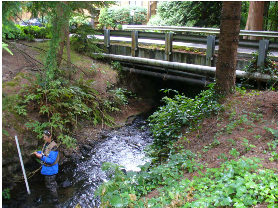
Photo 1: McAleer Creek bridge at Forest Creek Apartments
