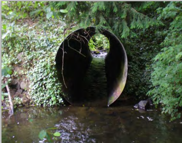
Photo 4. Forest Park Drive NE Culvert
