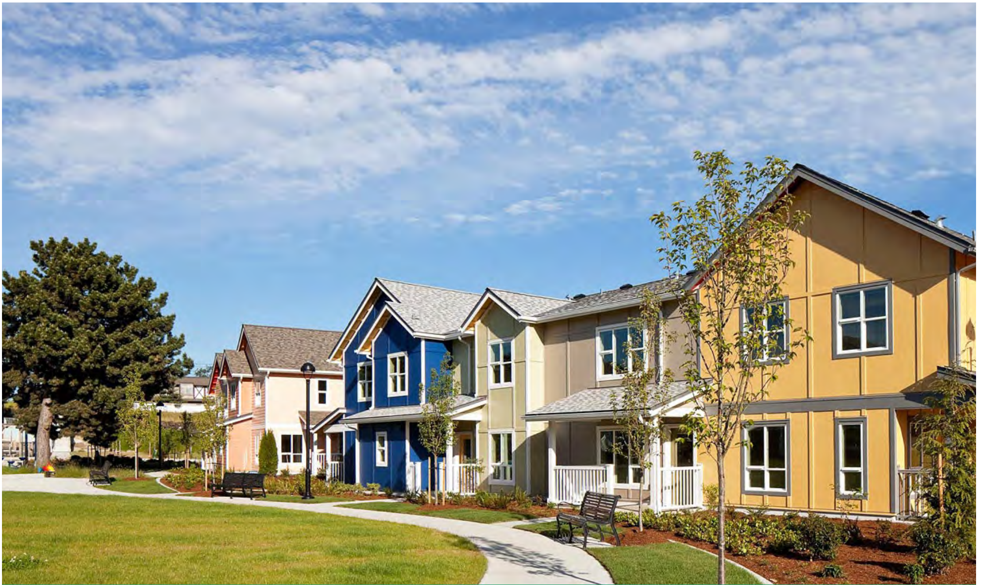
Affordable housing in Bend, Oregon
