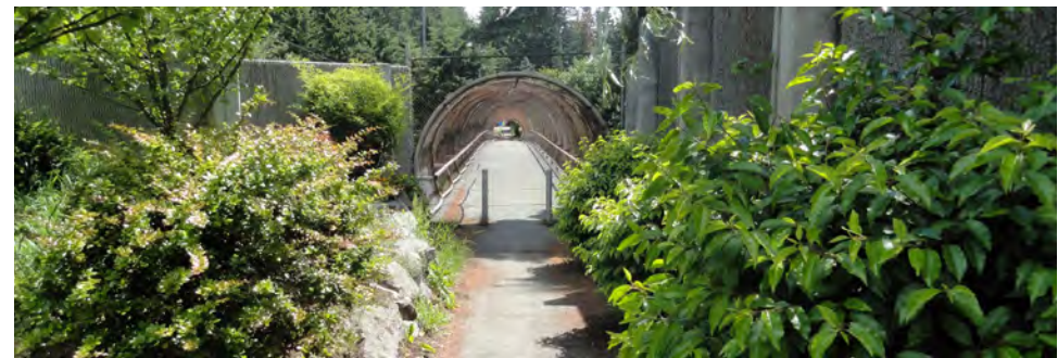
195th Pedestrian Bridge
