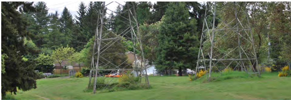
Seattle City Light Corridor
