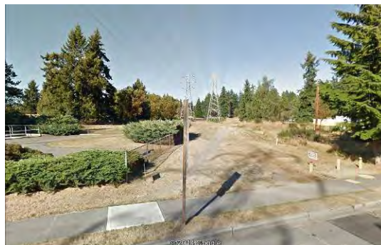
Seattle City Light powerline corridor
