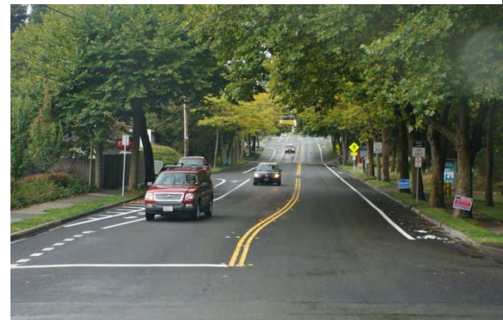
Recently completed bicycle lanes along NE 185 th Street
