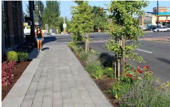
Aurora Avenue North green street improvements
