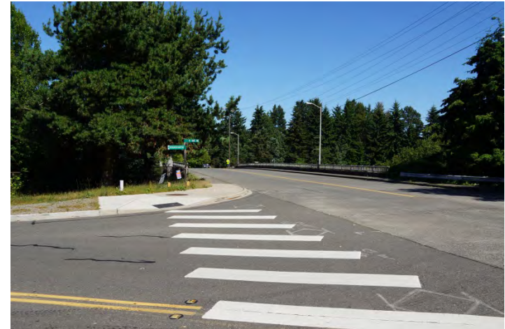
Current pedestrian facilities approaching the NE 185 th Street bridge from the west
