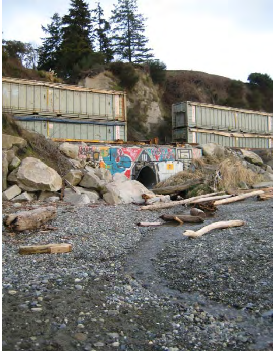
Photo 2. Culvert under BNSF railroad, mouth of Storm Creek
