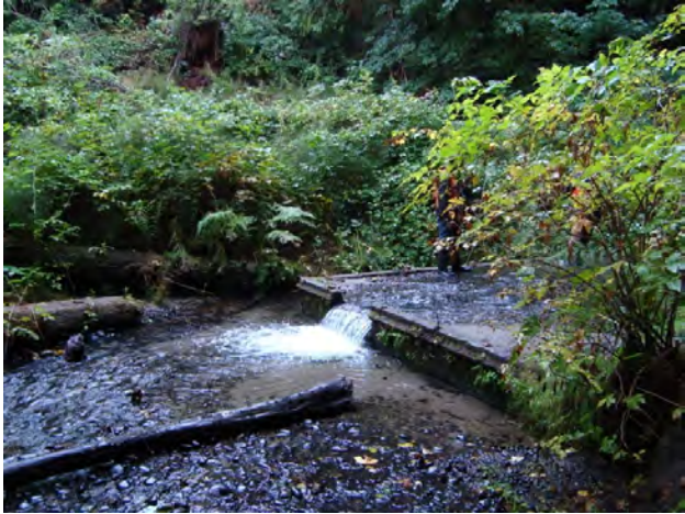
Photo 8. Concrete weir above Hidden Lake
