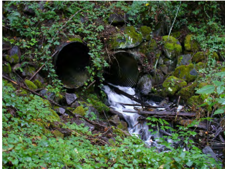
Photo 18. Culverts under NW Innis Arden Way
