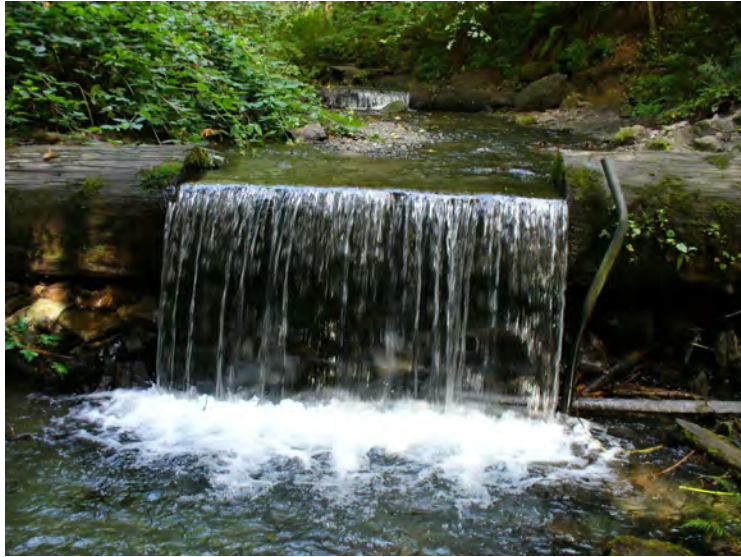
Photo 20. Channel downcutting below placed log weirs upstream of Hidden Lake; potential migration barriers at certain flow conditions
