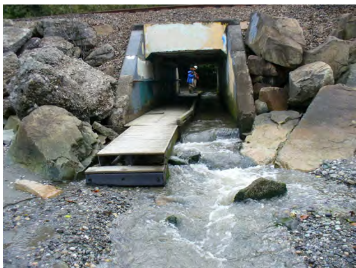
Photo 14. BNSF box culvert at the mouth of Boeing Creek
