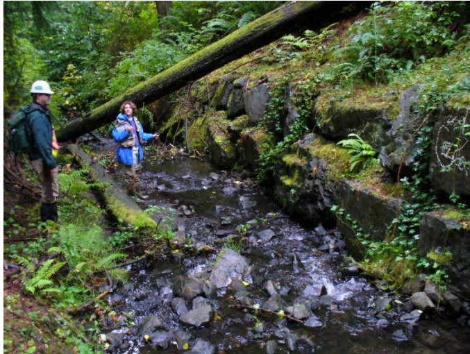
Photo 11. Stabilizing wall adjacent to right bank of North Fork Boeing Creek
