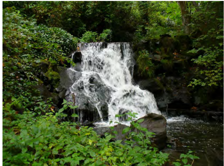
Photo 16. Grouted riprap cascade upstream of sheet pile dam
