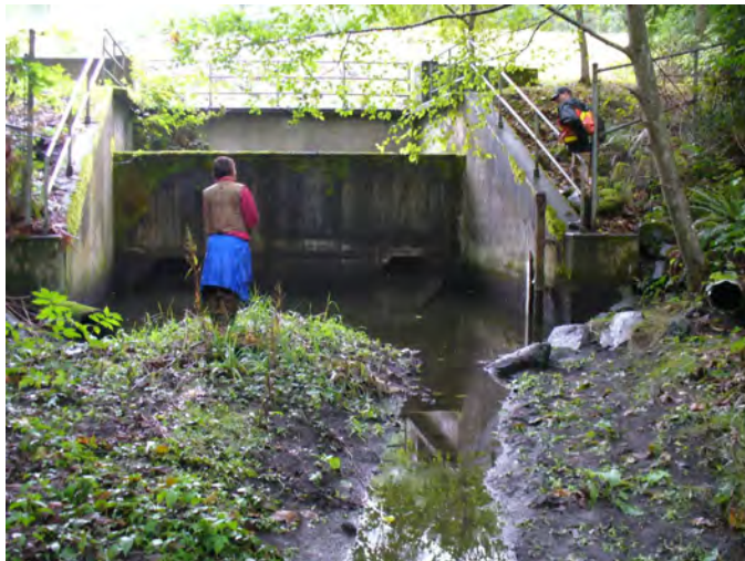
Photo 21. M1 dam outlet on South Fork Boeing Creek.
