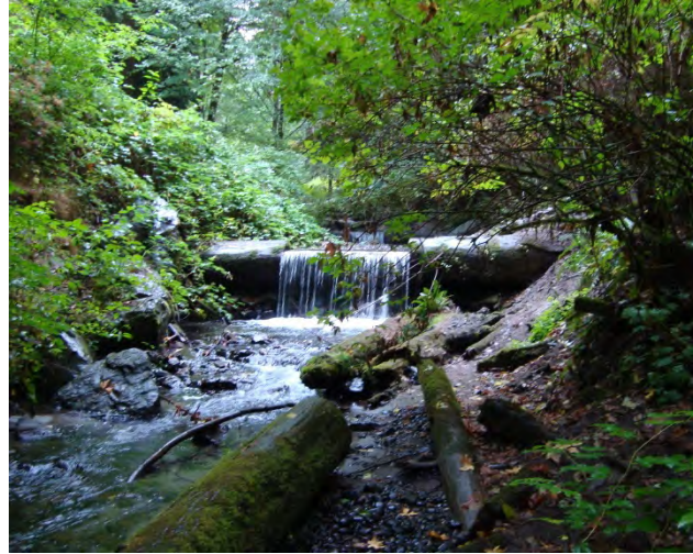
Photo 9. Example of typical log weir through Hidden Lake and Boeing Creek Park and North Fork reaches
