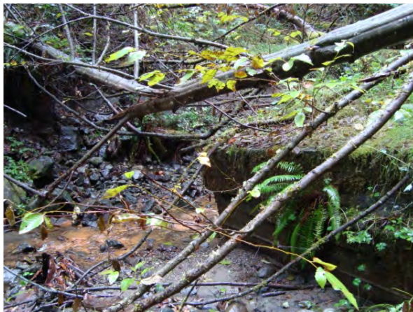
Photo 12. Concrete debris and oxidation in South Fork reach.
