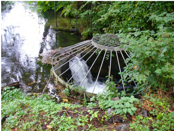
Photo 19. Hidden Lake dam and outfall control structure with trash rack
