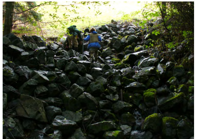
Photo 22. North Fork Boeing Creek detention facility outfall downstream of dam
