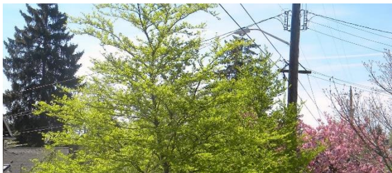
Tree growing into a power line.
